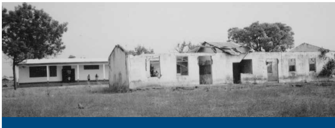
THE STORY OF KITOIE IS TOLD IN ITS TWO SCHOOL HOUSES – THE OLD ONE DESTROYED IN THE VIOLENCE OF 1992, AND A NEW ONE BUILT OUT OF A RENEWED SPIRIT OF TRUST BETWEEN THE GONJA AND KONKOMBA PEOPLE.
